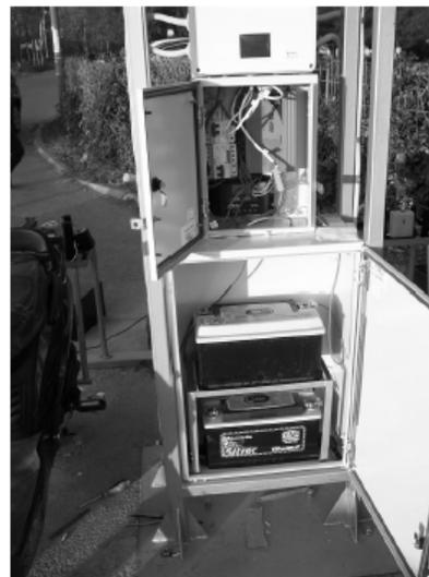
Figure 10. The panel of controller and batteries
