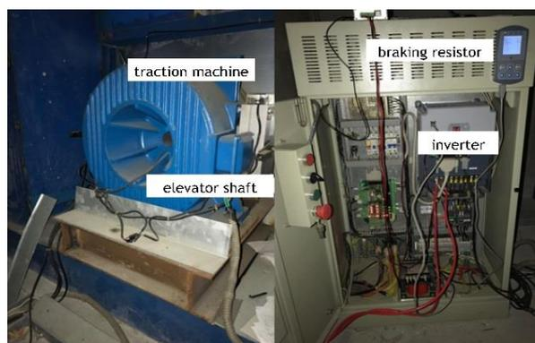
Figure 6. Elevator traction machine
